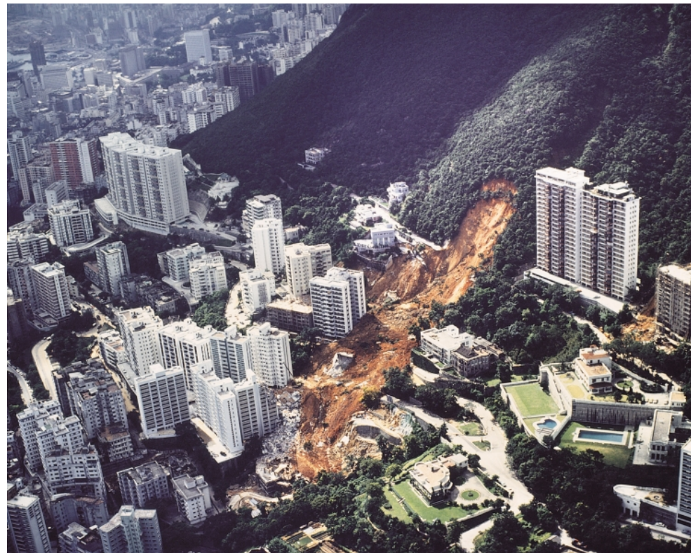
Po Shan Road Landslide, Hong Kong, 18.06.1972, www.hkss.cedd.gov.hk
